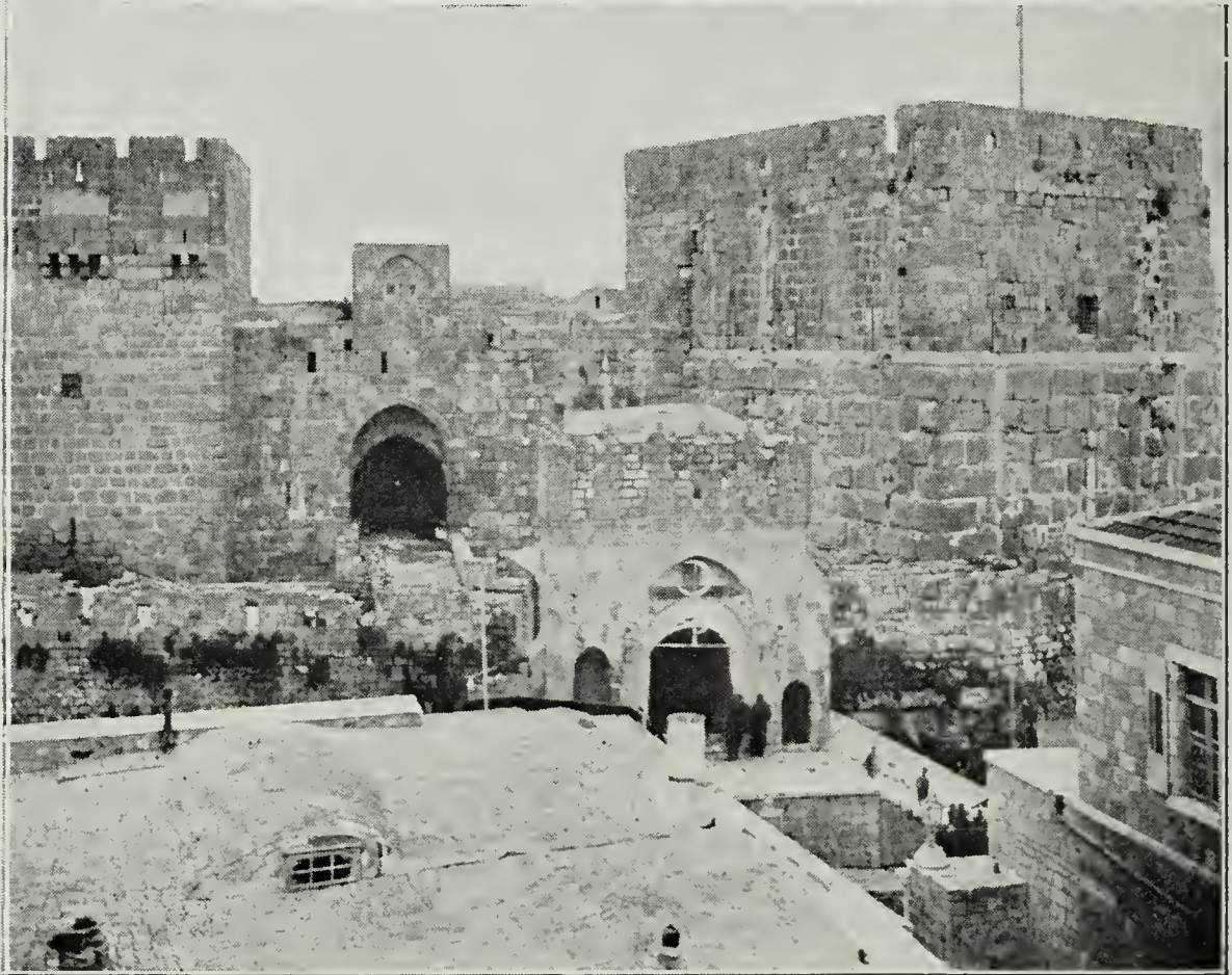
DRAWING SHOWING EXISTING REMAINS OF JERUSALEM AS IT WAS IN THE TIME OF CHRIST.
